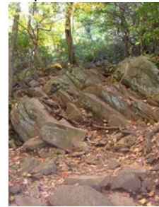
B26 – Eroded diabase columns
