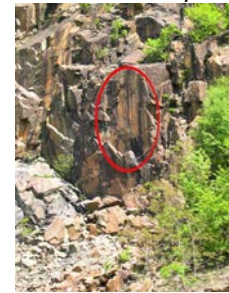
V10 – Colossal plume on Quarry wall
